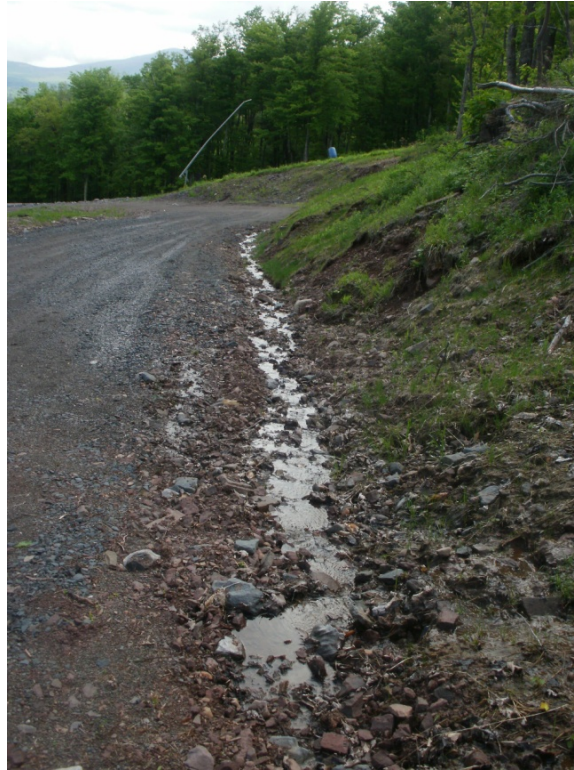
PHOTO 1: Water flowing in rock lined ditch (1-2 gpm) along unfinished road in the development west of Ski Windham at approximately 2,500 ft elevation.
