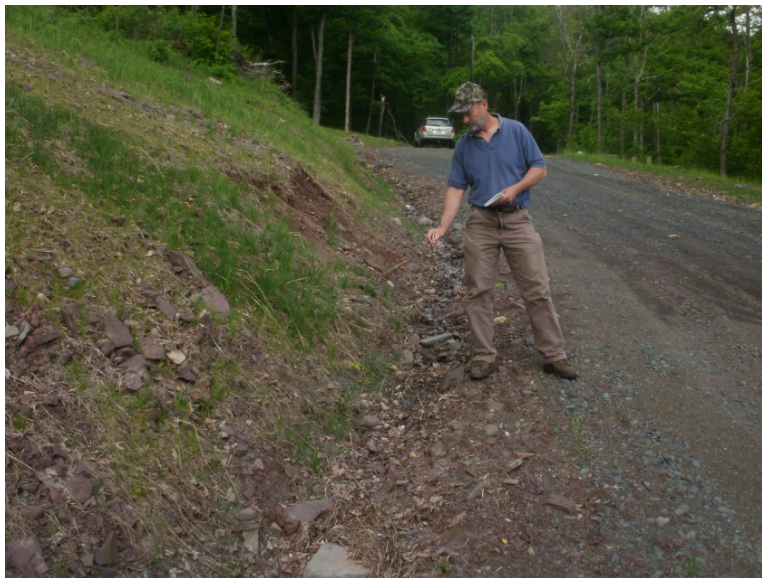
PHOTO 2: All of the flow seen in Photo 1 has infiltrated the subsurface by approximately 200 feet from where the flow originated.
