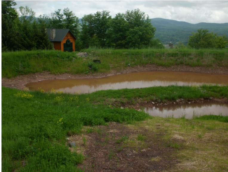
PHOTO 3: Low water level in retention pond on May 24, 2012, down slope from Photos 1 and 2, with no overflow or discharge two days after 1.5 inches of precipitation.
