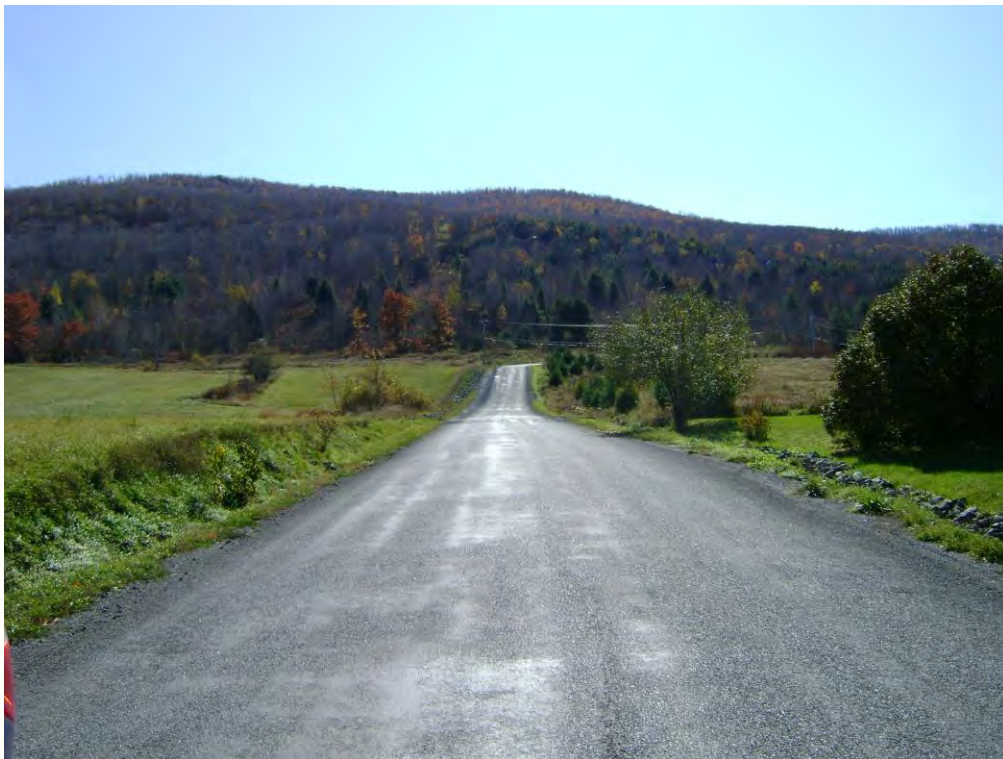
View south up Trailside from near South Street. The grade, or slope, of the section of road before the road curves to the right is approximately 13% for a length of 230 feet.
