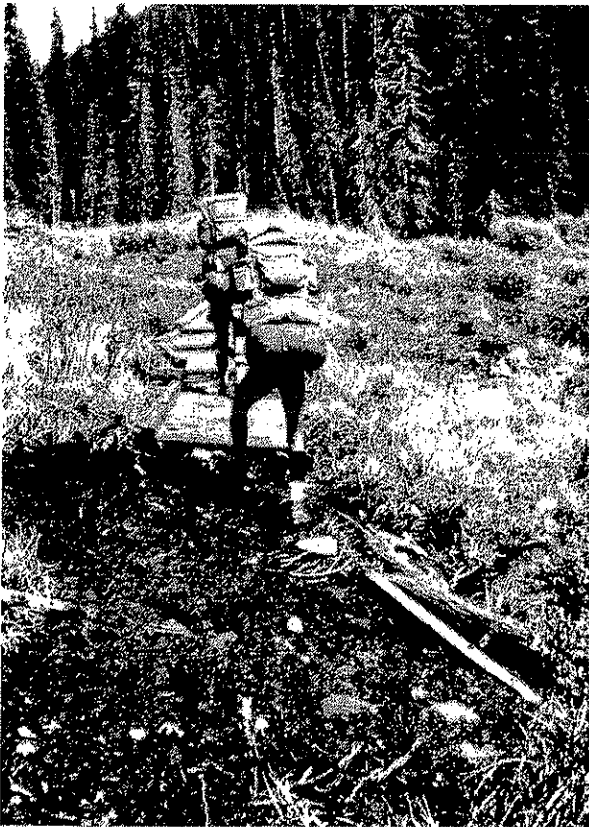
Fig. 15.18. Trails through areas of water-saturated soils develop into ever-larger bogs. In many cases the only solution is to bridge the area. It is best to bridge the entire bog, rather than just part of it—the problem with this trail. Photo courtesy of the USFS.
