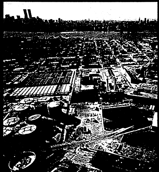
NEWTOWN CREEK WATER POLLUTION CONTROL PLANT
