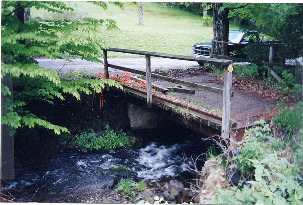
Photo 1. Bridge to Silo A, view north.
