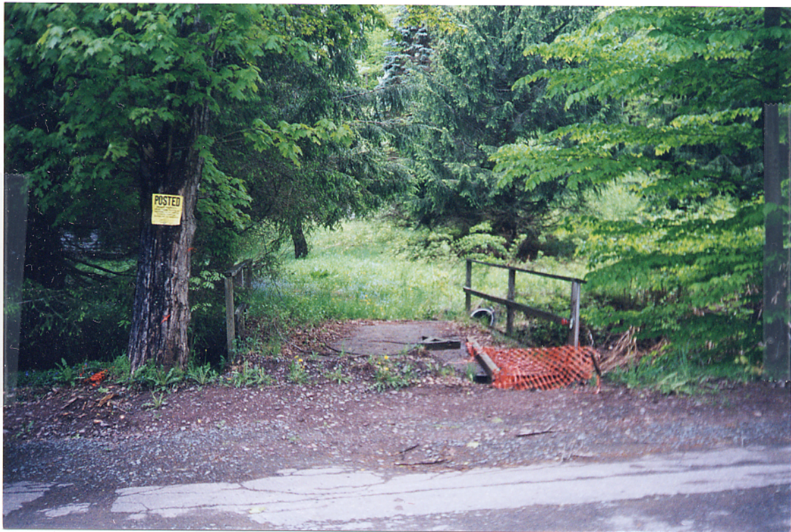
Photo 2. Bridge to Silo A, view south.
