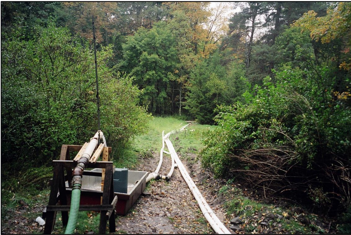
Photo 20. View from well K-2 towards well K-1, which is just out of site. Well K-3 is out of sight, just off to the right. (Photographed Sept. 2007.)
