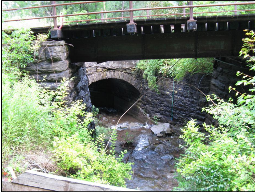
Photo 9. Todd Mountain Rd. Brook, viewed from south end of lines WA and WB, towards the railroad bridge and the road bridge (stone arch). The water supply line will be buried in the roadbed of Todd Mountain Road at that bridge. (Photographed July 30, 2009).
