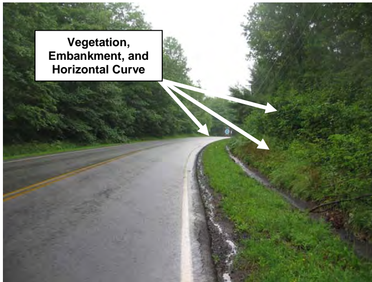
Photograph 2 – Sight Distance Looking Right (from edge of pavement)
