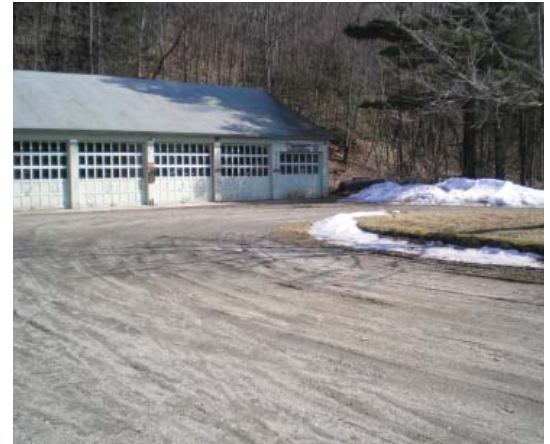
Green Mountain National Forest Workshop Rehabilitation
