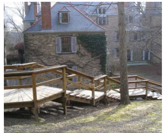
Grey Towers (Stair Reconstruction)
