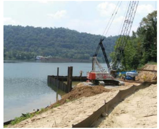
Wayne National Forest Boat Launch (under construction)
